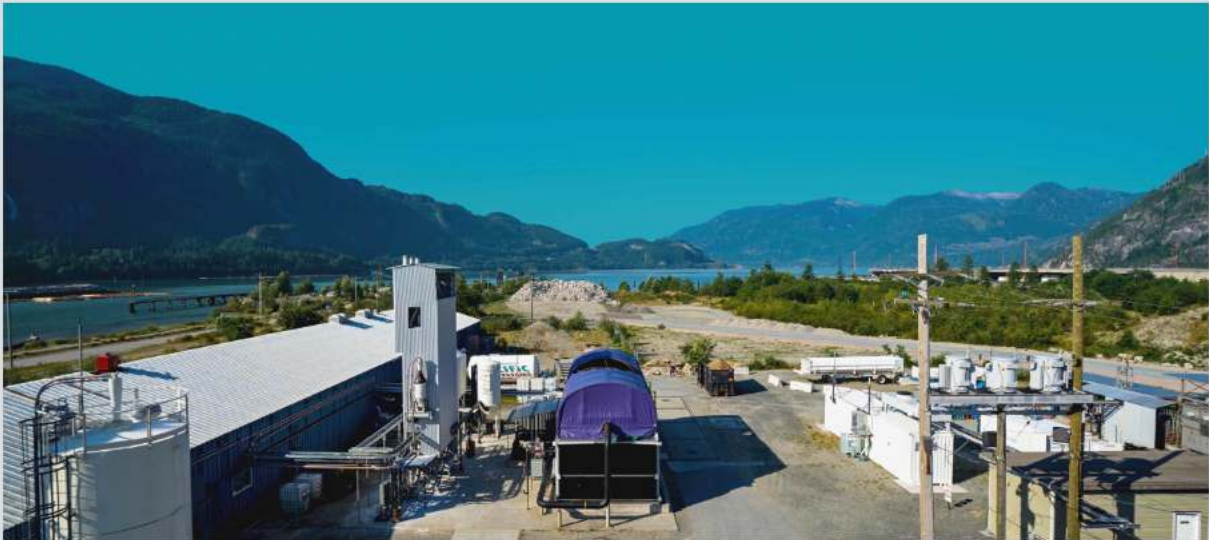
Carbon Engineering's Squamish, B.C. facility.
